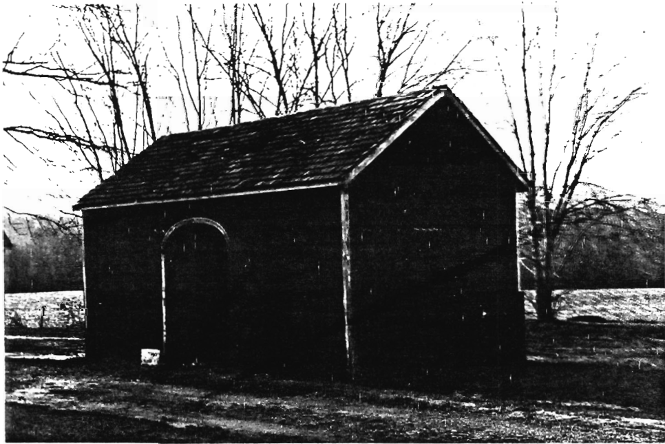
Stable C, view to SW.
