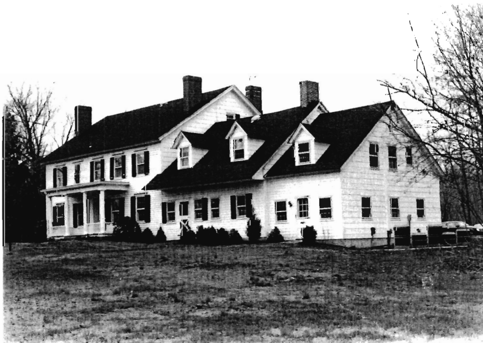
House (A), view northwest of main elevation. 1981 photograph.
