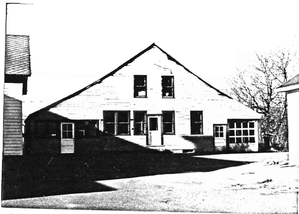
1328-3 (continued) Wagon shed, view to N.
