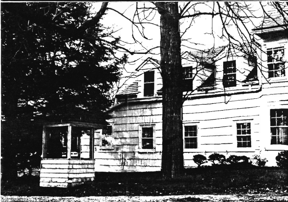
House, wing and well house, view to NW.
