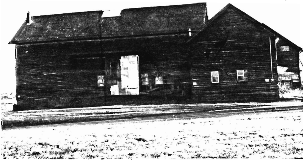
Barn Complex C, view to S.
