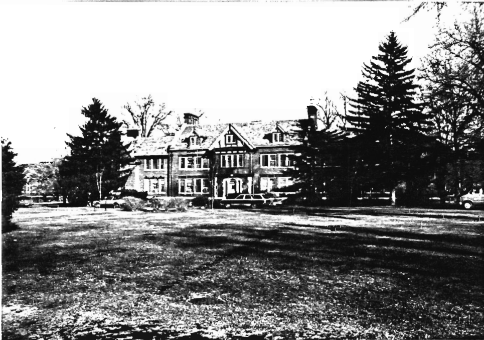
Building 14, view to NE.
