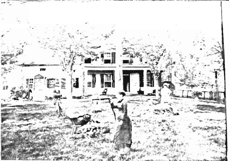
House, historic photo from late 19th-early 20th century. View to N.
