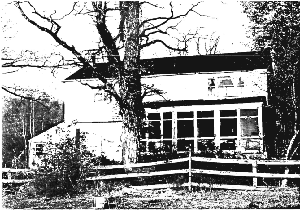
House A, view to N.
