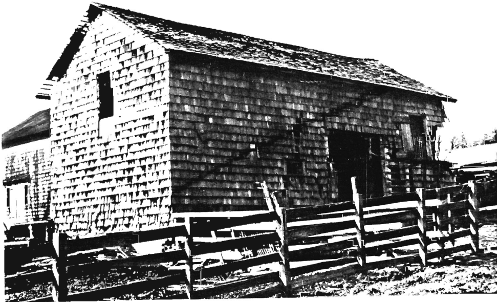
Small Barn C, view to NW.
