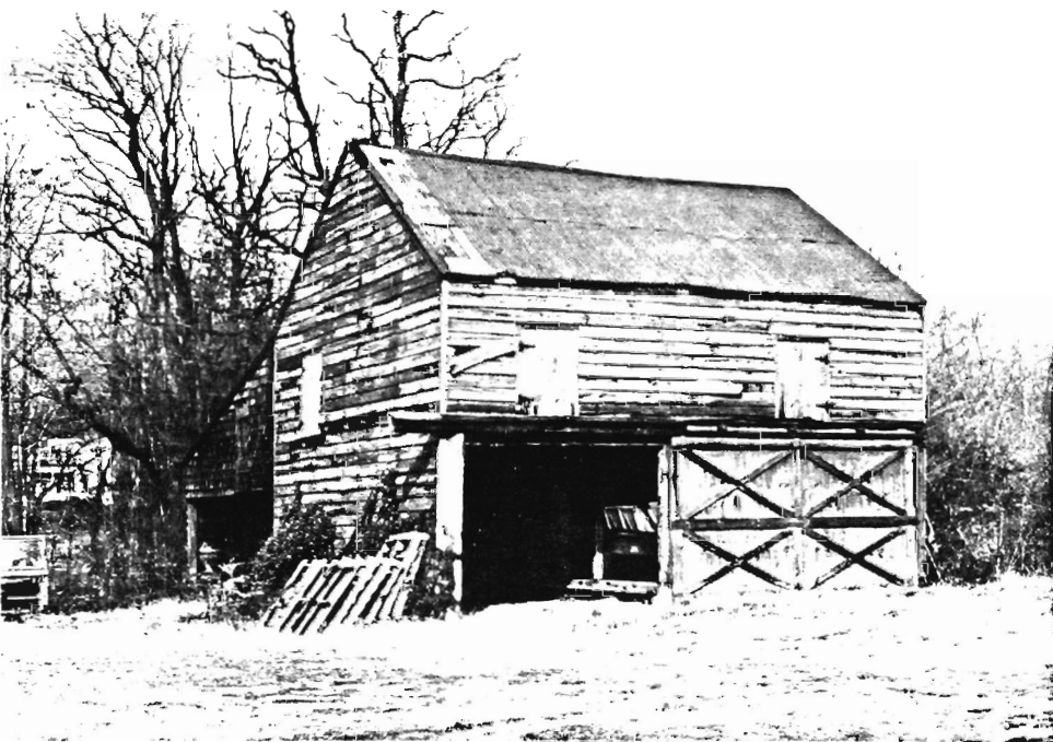
Wagon Shed, view to NE.
