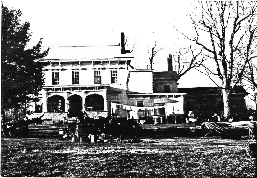
House A, view to N
