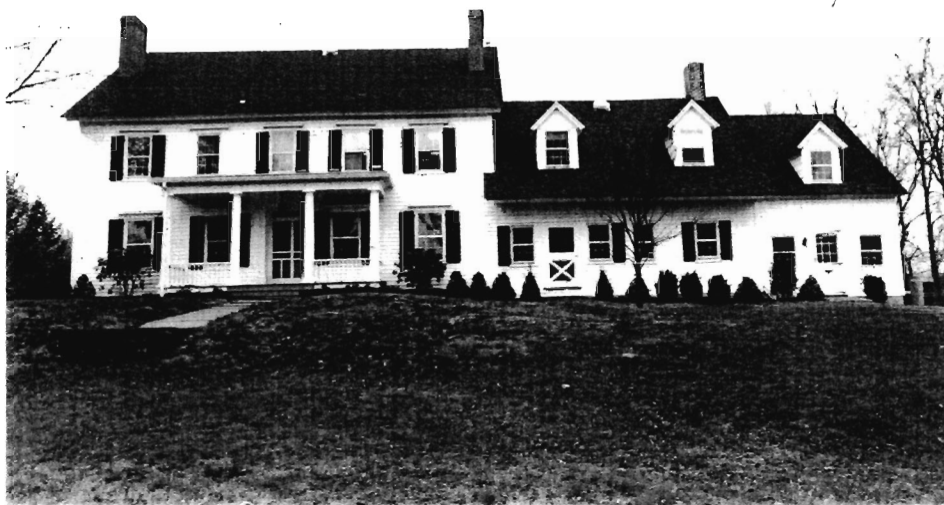
House (A), view north of main elevation. 1981 photograph.
