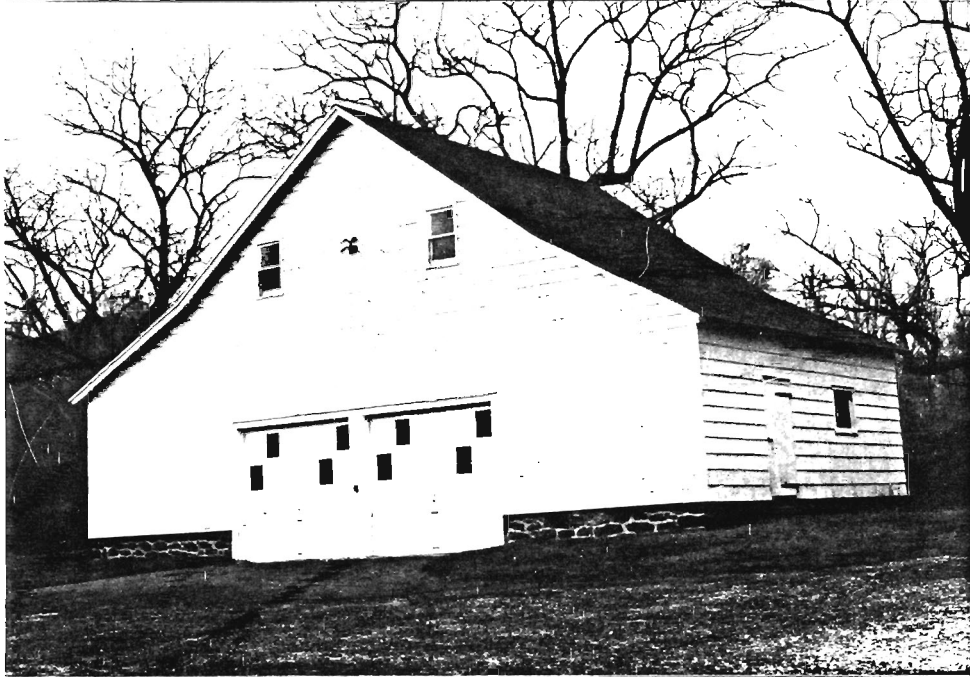
Wagon shed, view to NW.
