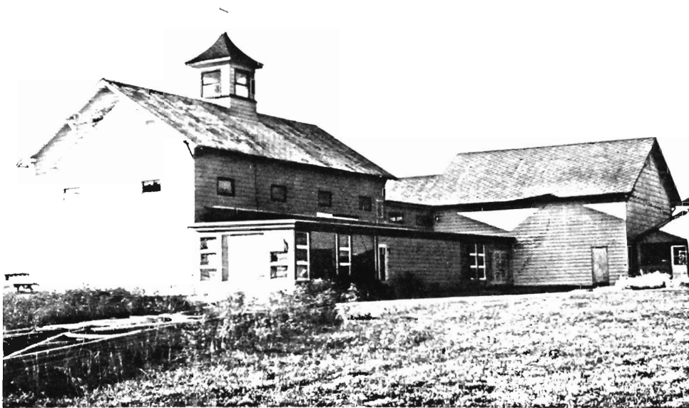
Barn complex, view to NW.
