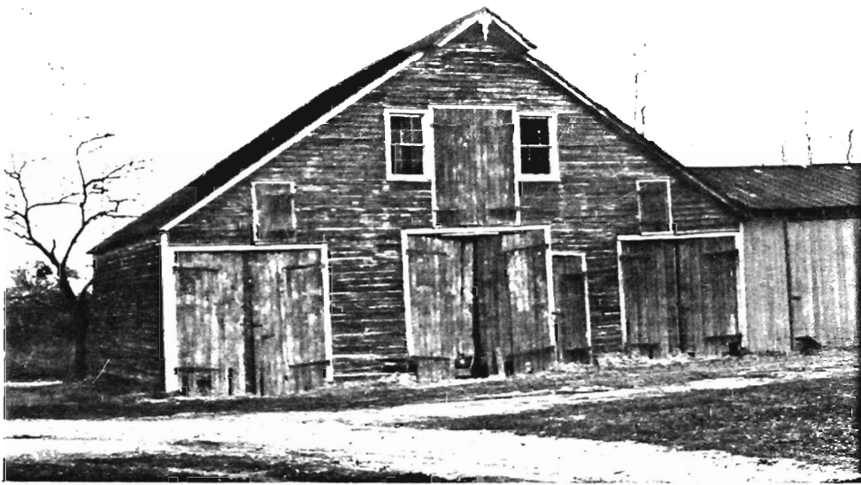
Wagon Shed B, view to NE.
