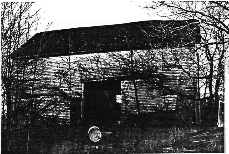
Barn C, view to N.
