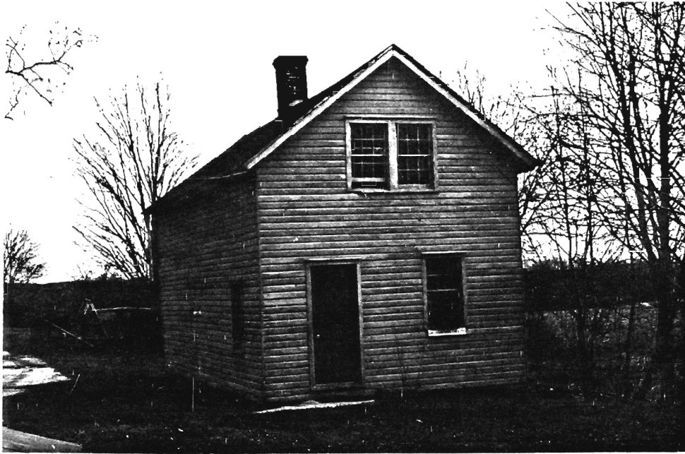
Tenant House, view to SE.
