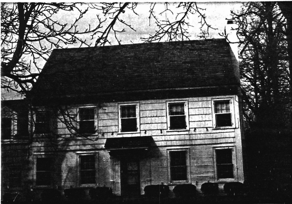
House, main block, view to N.
