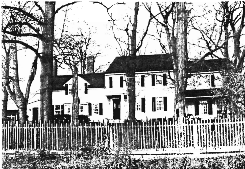
House A, view to N.
