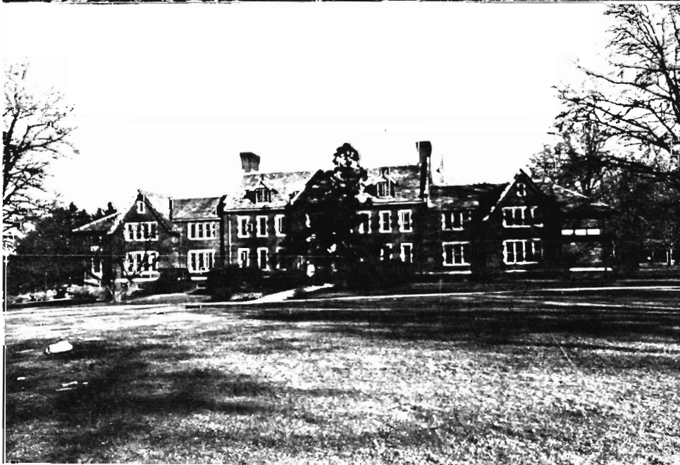
Building J, view to NE.
