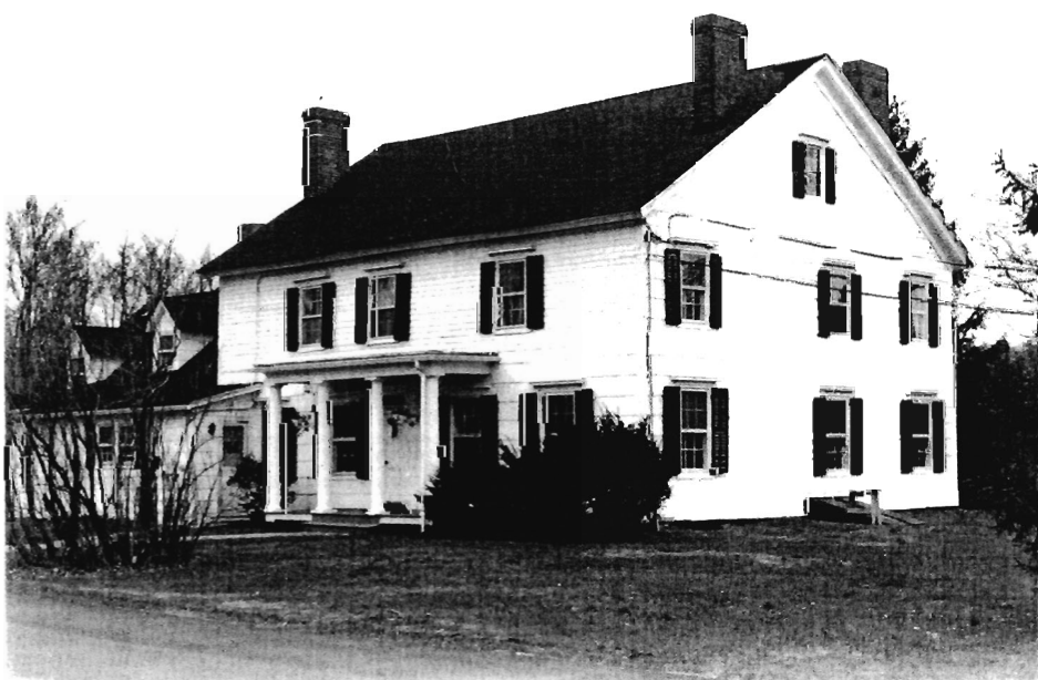
House (A), view southeast of rear elevation. 1981 photograph.
