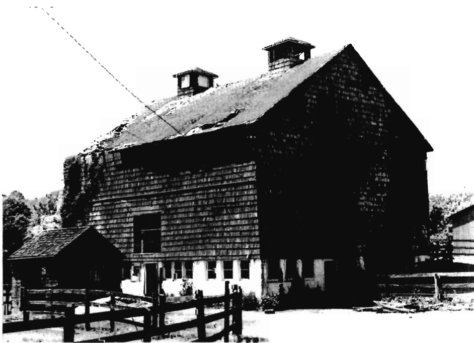
Barn (B), view northwest. 1992 photograph.
