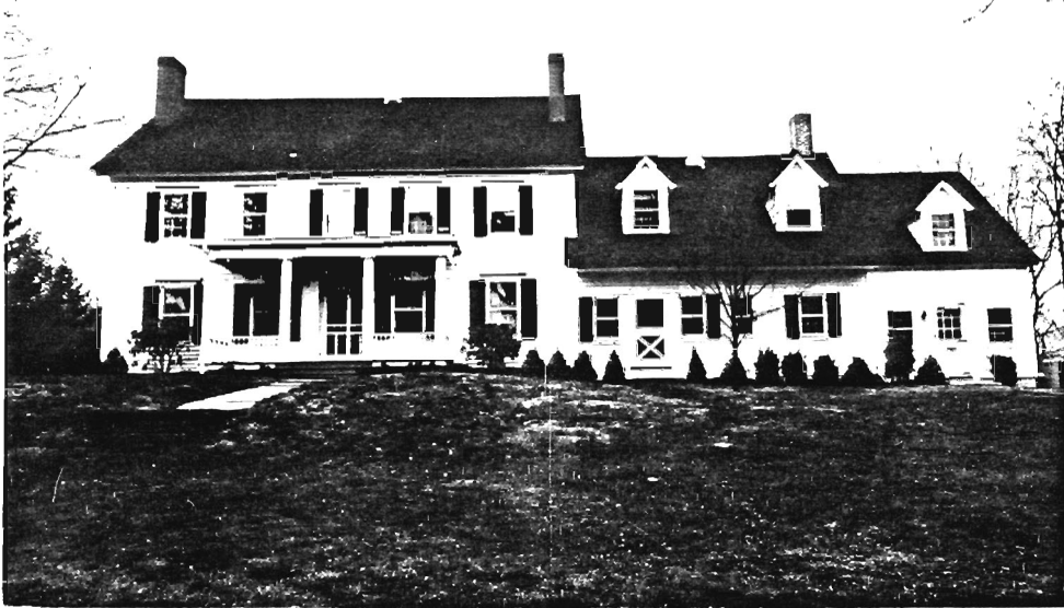
House A, view to N.
