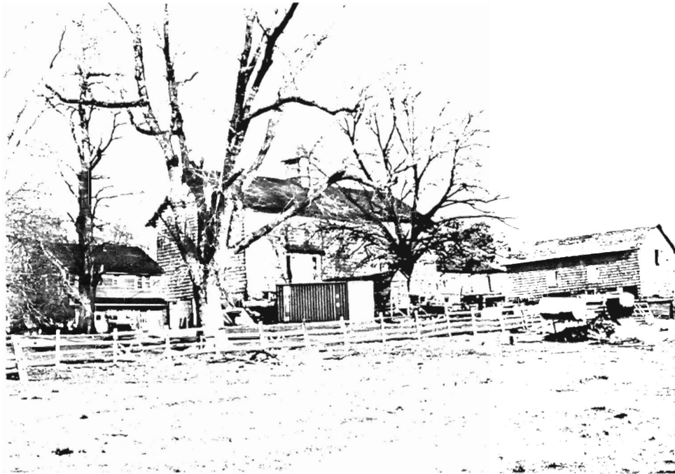
Barn Complex, Large Barn B and Small Barn C, view to NE.
